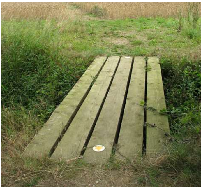
Figure 27 – Example of suitable plank footbridge across channel
