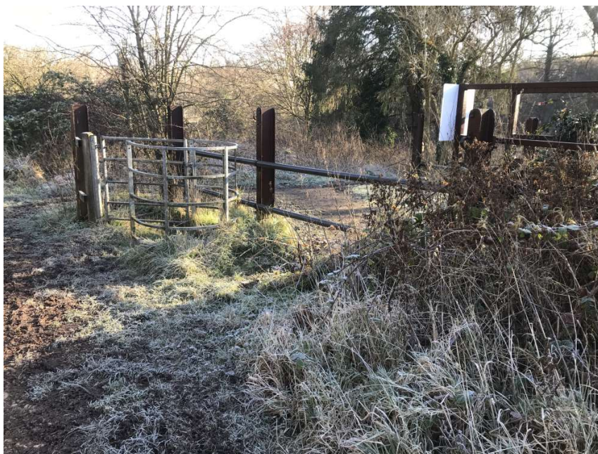
Figure 31 – Redundant gates and metalwork at entrance D to be removed
