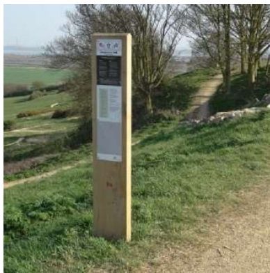
Figure 22 Example simple marker post for tertiary entrances
