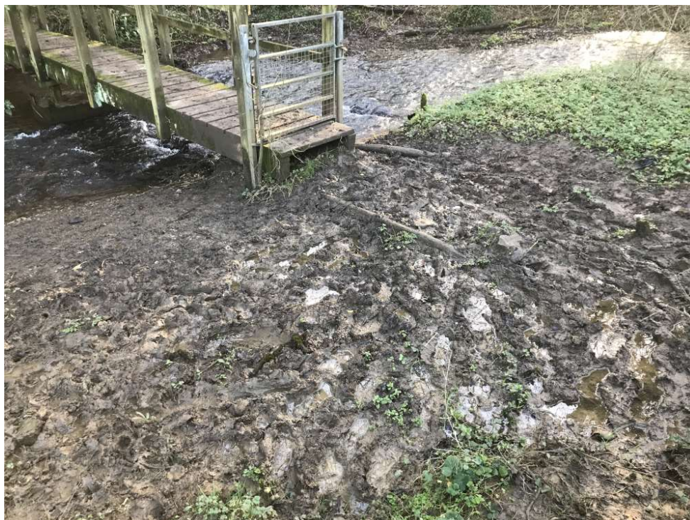
Figure 15 – Extreme level of mud by footbridge near entrance H
