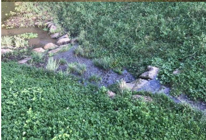
Figure 28 – Example treatment for channel with boulders forming weirs and small pools behind
