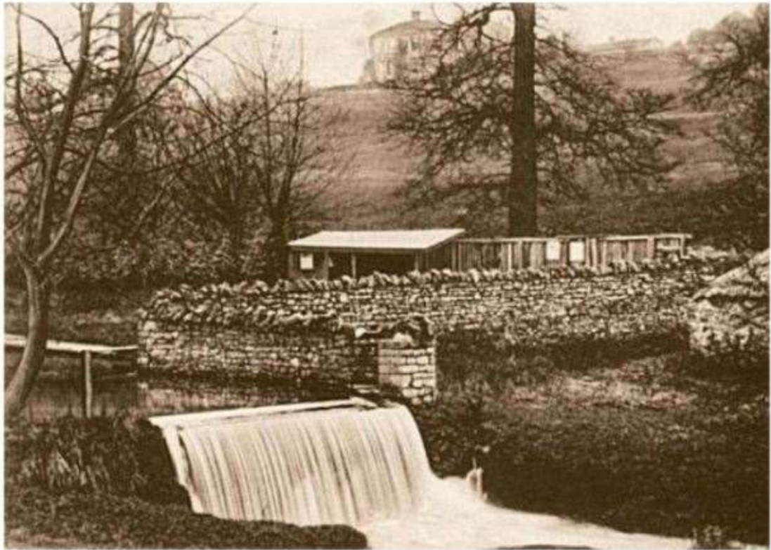
Figure 4 – Miners pool, postcard image possibly c.1907. Note South Hill House on the ridge, where Bath College now stands
