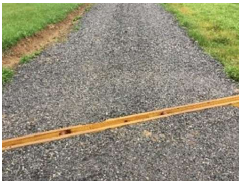
Figure 24 – Example of timber drainage cut off
